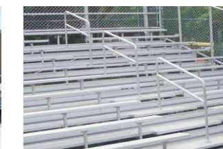
Handrail for middle aisle
